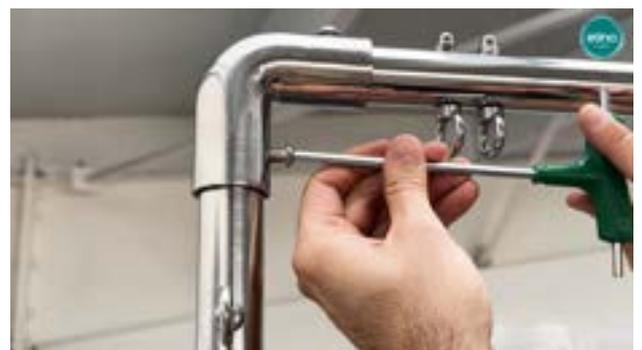
We insert the long bars into the metal structures that we have hooped and then we place and screw the upper metal structure that acts as a bridge.
